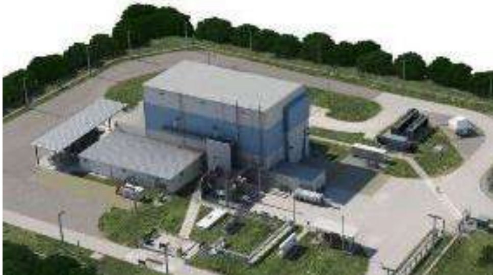
Figure 7-4. Multi Payload Processing Facility (MPPF)
