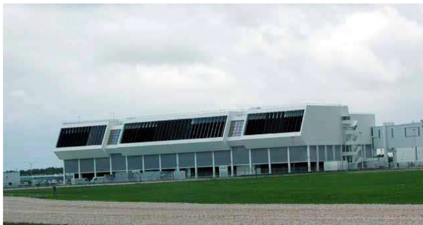
Figure 7-13. Launch Control Center
