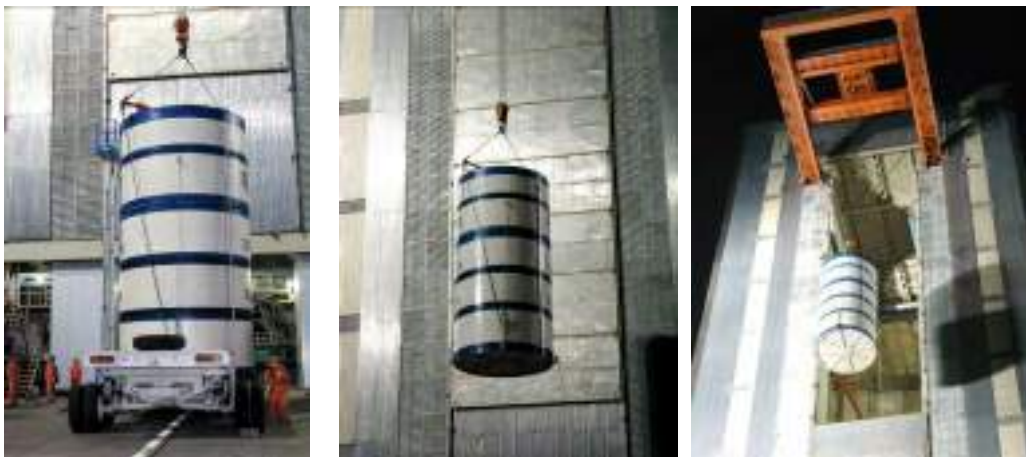
Figure 8-6 SC Container Lift
