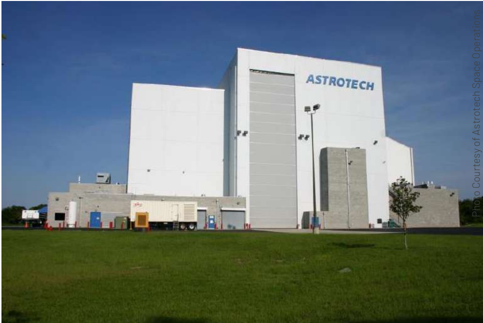
Figure 8-4: PPF at Astrotech Space Operations – Building 9
