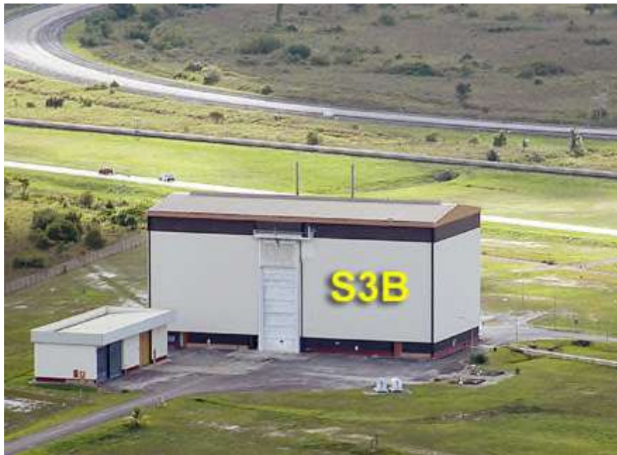
Figure 6.2.2.2.b – S3 area overview
