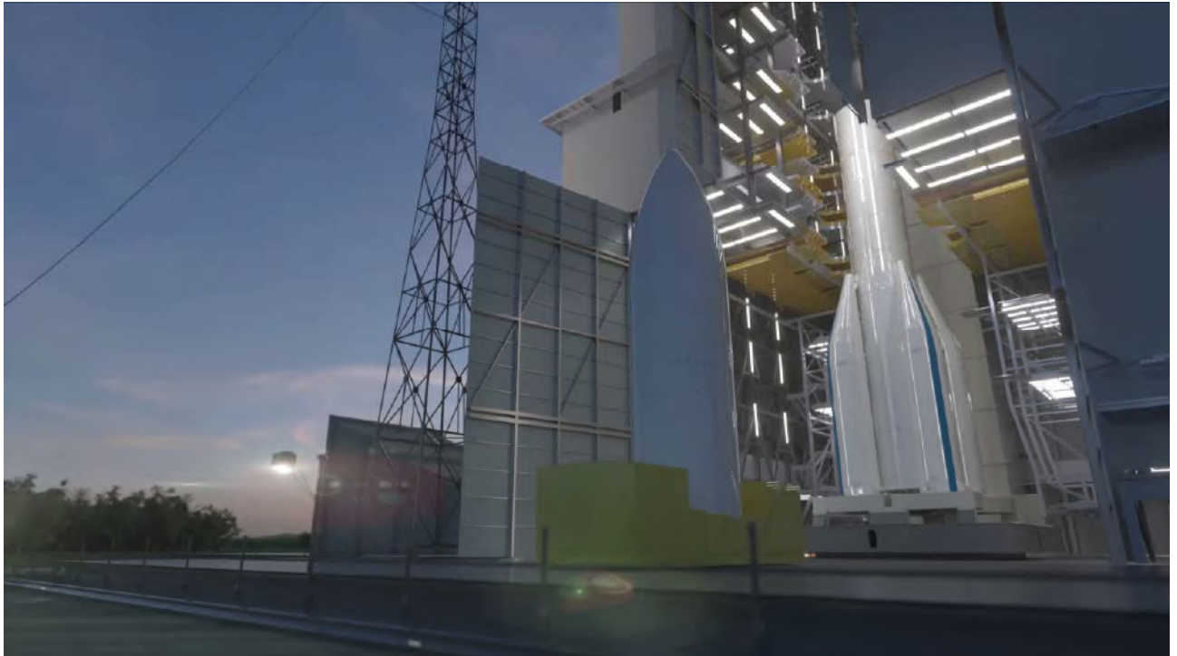
Figure 6.2.3.2.1b – Arrival of upper composite in the mobile gantry
