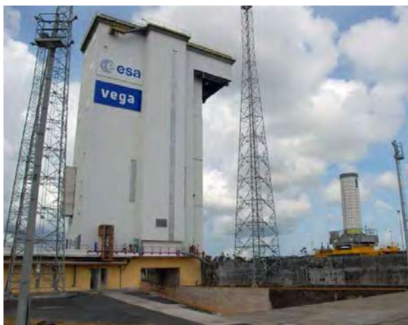
Figure 6.2.3.2.1c – Transporter arrival in front of the mobile gantry, which is positioned over the launch pad
