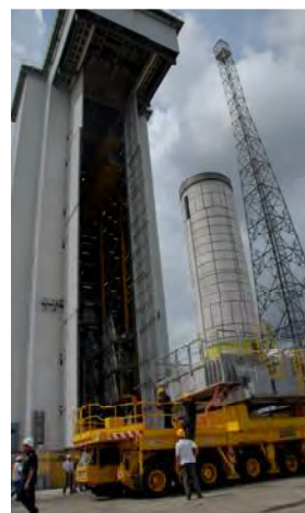
Figure 6.2.3.2.1d – Transfer of the P80 first stage atop its pallet onto the launch pad through the gantry's open doors.
