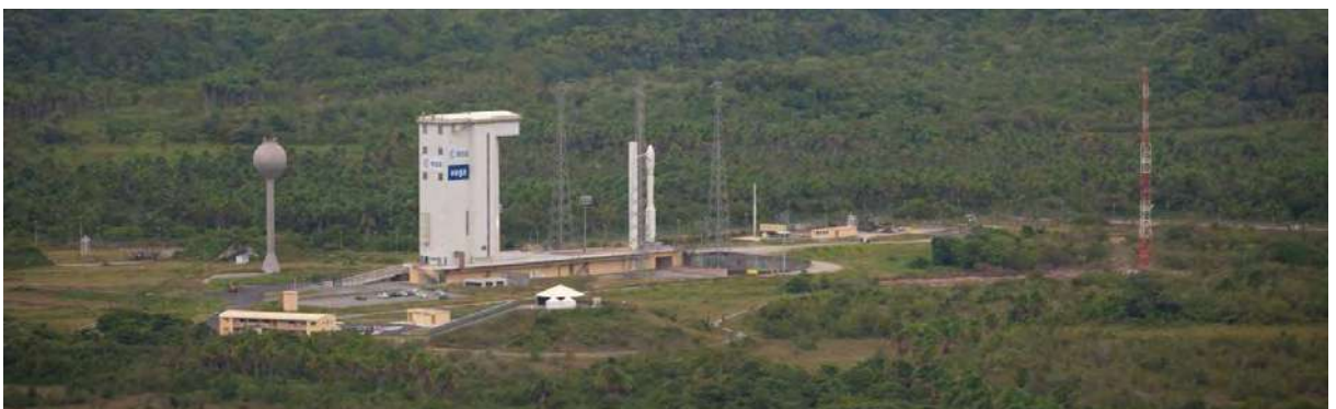
Figure 6.2.3.2c – Vega launch site – Water tower on the left
