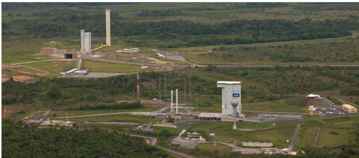
Figure 6.2.3.2.1r – Vega launch vehicle ready for final launch preparation sequence
