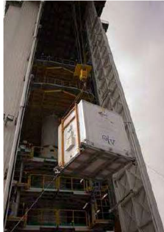
Figure 6.2.3.2.1k – Arrival of the AVUM upper stage in its container, and hoisting to the upper platform inside the mobile gantry
