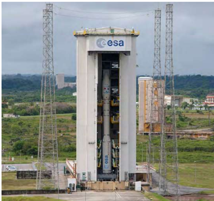
Figure 6.2.3.2.1q – Mobile gantry roll-back
