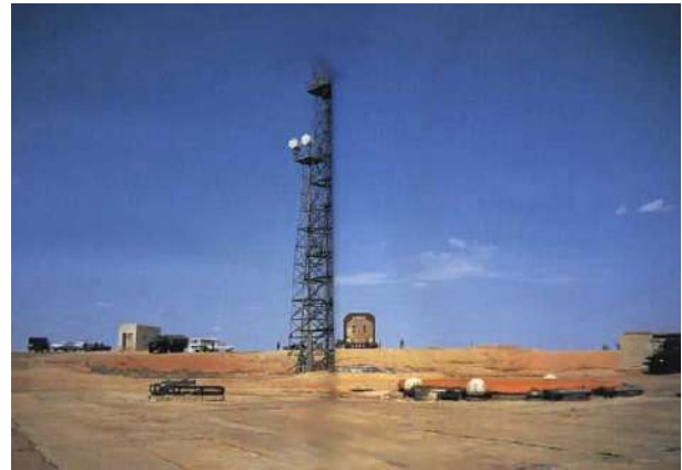
Figure 6.4-1 Dnepr Launch Complex Facilities (Sites 106 and 109)
