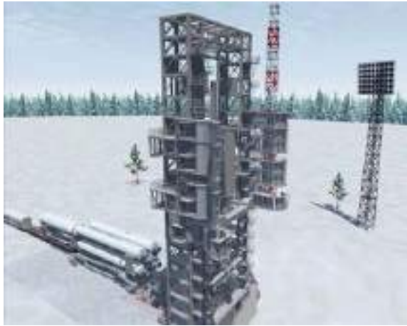
Figure 1.10.3-1: Transporting Angara A5 LV to the Universal Launch Complex and Erecting on Launch Pad
