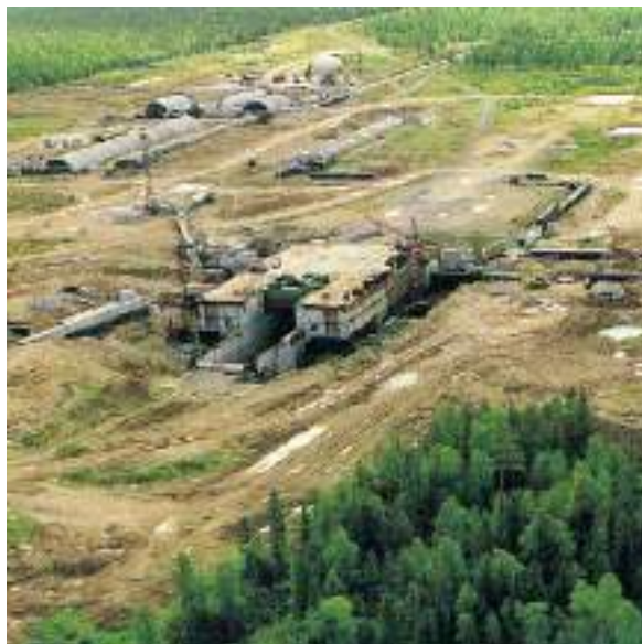
Figure 1.10.2-2: Construction of Universal Launch Complex
