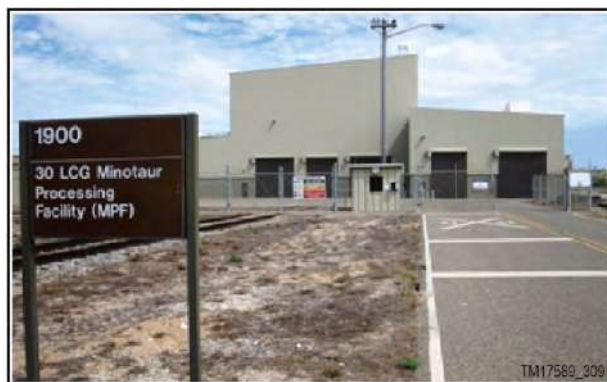
Figure 7.1.5-1. Minotaur Processing Is Performed at the MPF at VAFB
