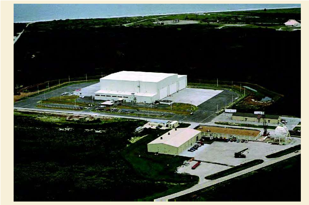
Figure 7-16. Space Launch Complex 37, Horizontal Integration Facility—Aerial View
