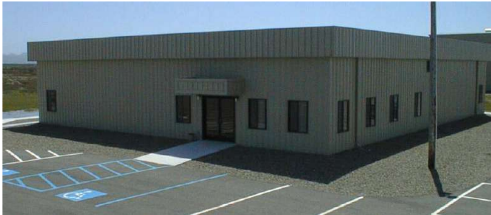
Figure 7.2.1.1-2: Technical Support Building
