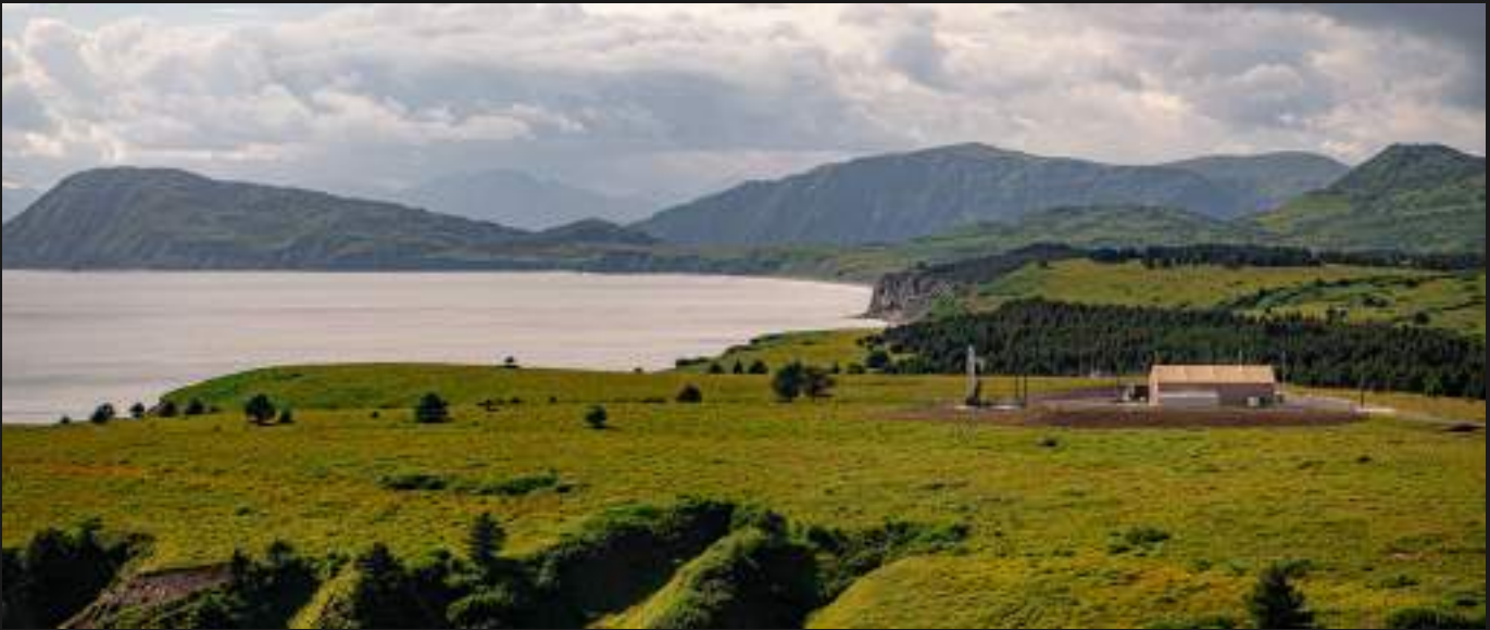
FIGURE 17. PAD B AT PACIFIC SPACEPORT COMPLEX - KODIAK, ALASKA
