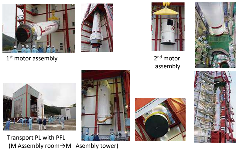
Figure 5.1.3-4 LV Assembly in M Assembly Tower
